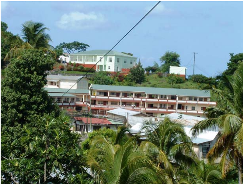
St. Rose Convent (background) and St. Rose Modern Secondary School (middle) after repair and reconstruction from Hurricane Ivan.
